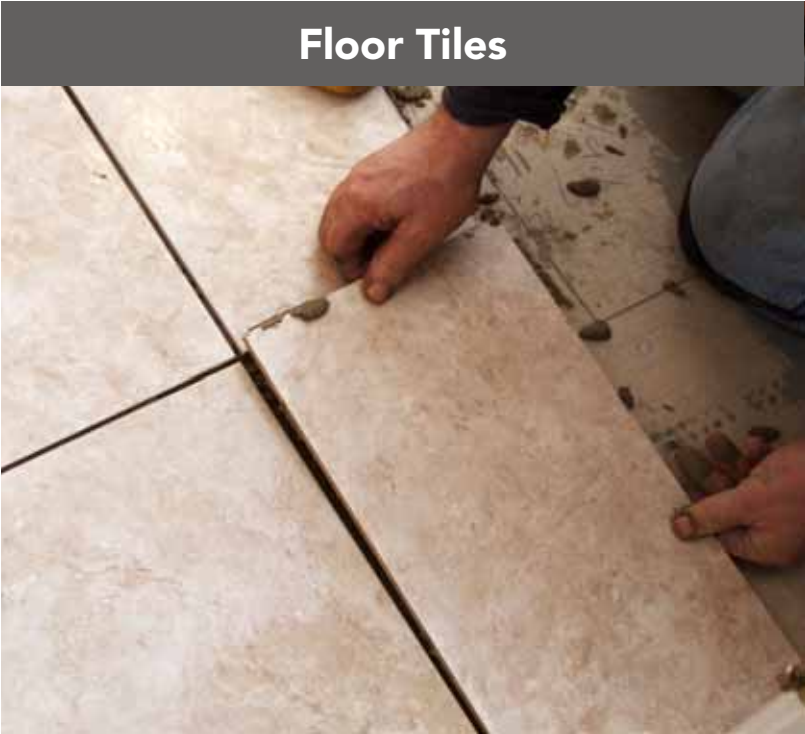
We lay the floor tiles before we install the interior trim. Then the drywall is checked, the fireplace installed and the interior paint completed. This is the last step before we move on to the kitchen and vanities.
