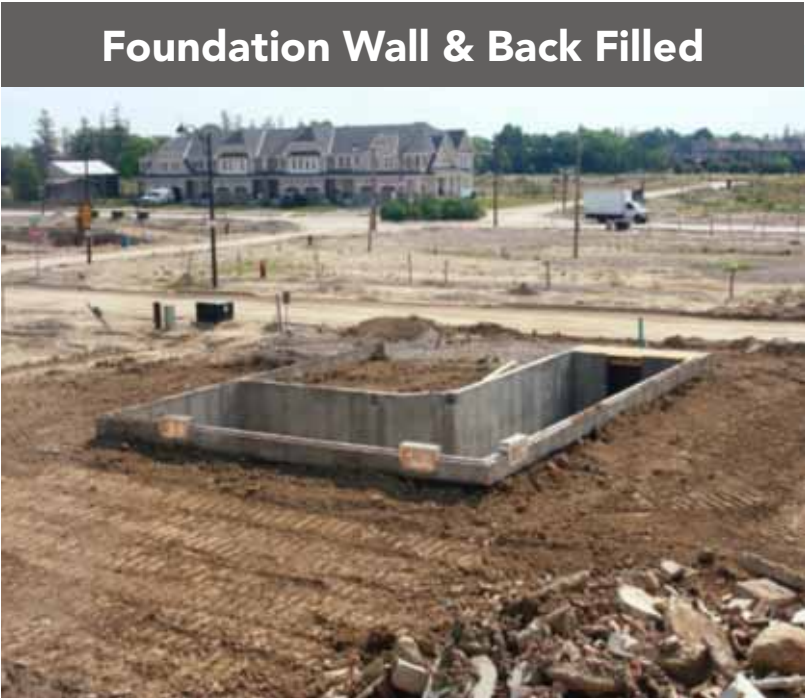
Prior to the backfill of your foundation, the Municipality conducts a back-fill inspection to ensure that the foundation weeper system is installed in accordance to OBC standards.
